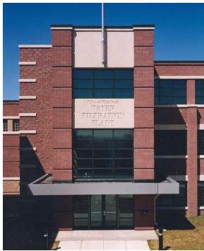
Oshkosh's Water Filtration Plant constructed in 1999
